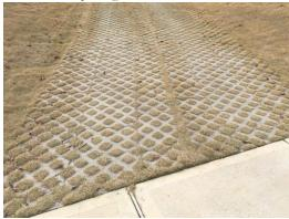
**Biofiltration Strip**-water velocity is decreased as well as the amount of runoff.
