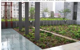
**Bioretention-**water flows into an area, is treated and infiltrates into the ground decreasing stormwater volume.
